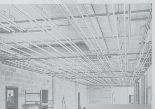
Figure 50. Ceiling Showing Heating and Electrical Conduits (Complete Room)
