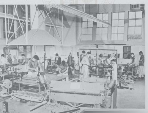
Metal Laboratory (Figure 79). This junior high school metal laboratory with smaller equipment shows an excellent use of safety lines to determine operator areas.
