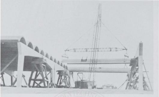
Figure 41. Erection of Concrete Shells
