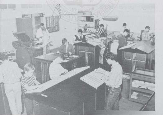
**Graphic Arts Laboratory** (Figure 83). A junior high school graphic arts class in action showing compositing work in progress, a student locking up a chase, and the instructor checking the alignment of a job on the press.
