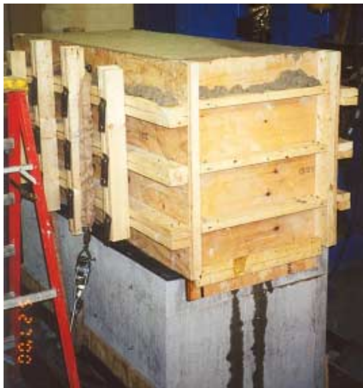
Figure 4.4. Pictures from construction of the revised VDOT semi integral abutment hinge
