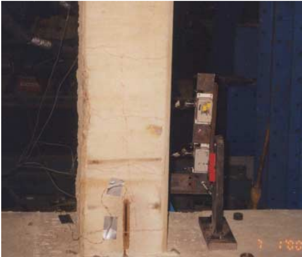
Figure 5.24. Progressively developed tension cracks in concrete pile
