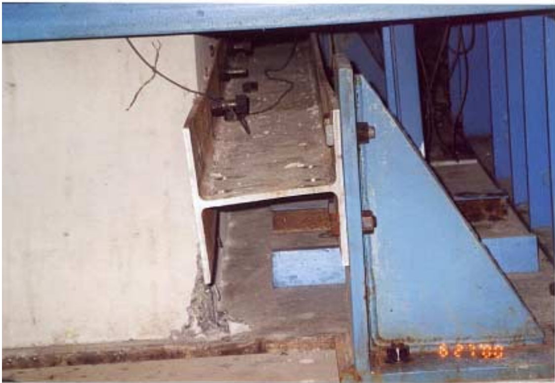
Figure 5.3. Mounting pile caps to reaction floor by L-shaped steel elements
