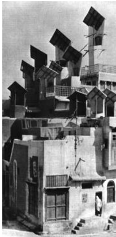
14. Rooftop wind scoops, Sind District, West Pakistan In use since 1,500 a.d.
