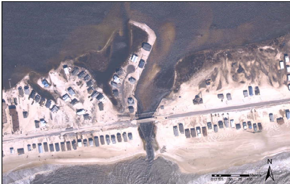
Figure 4-36 (Little Lagoon Pass in 2004, damaged by Hurricane Ivan)
