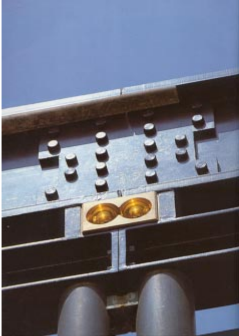
Detail of connectors for colonettes and of the trabeation: loggia on the Banca Popolare, Verona
