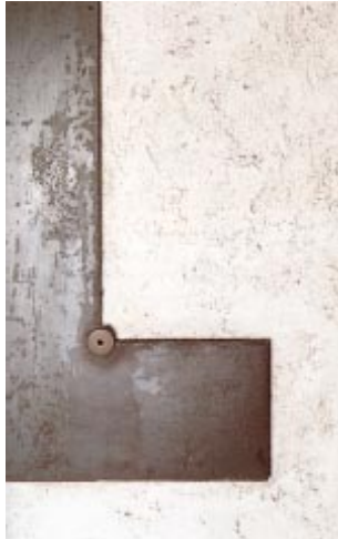
a Detail of profiling in iron on a passage of the Castelvecchio Museum, Verona.
