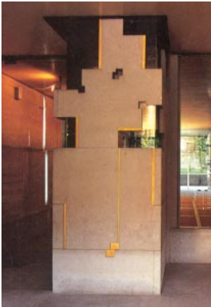
Column at Quarini Stampalia
