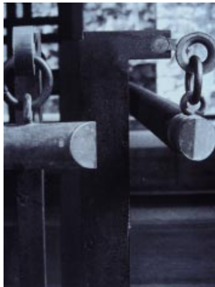
Detail of barrier in the Castelvecchio Museum, Verona
