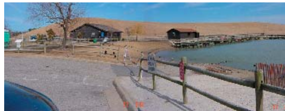
view from parking lot up to landfill
