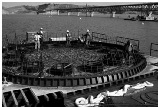
Figure 3: Pier 3 of the third Four Bears Bridge in 2004 (NDDOT, 2005)
