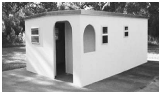
Figure 1. Small House Built Using Sandwich Composites (DuraSip, 2009)
