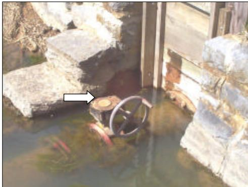
The next step in starting up the mill is to open the gate valve at the dam. This valve located on the face of the dam controls the flow of water to the mill. During times when the mill is not operating a small amount of water is allowed to flow in order to keep the water wheel turning for esthetic purposes only. The water wheel is not connected to the stones. The setting of the gate valve (arrow) for these circumstances is no more than 1/8 open.
