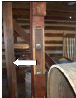
The engaging of this gear will then turn a vertical shaft going to the third level (arrow at left). This shaft then powers the head of the elevator leg, as well as the bolting reel.
