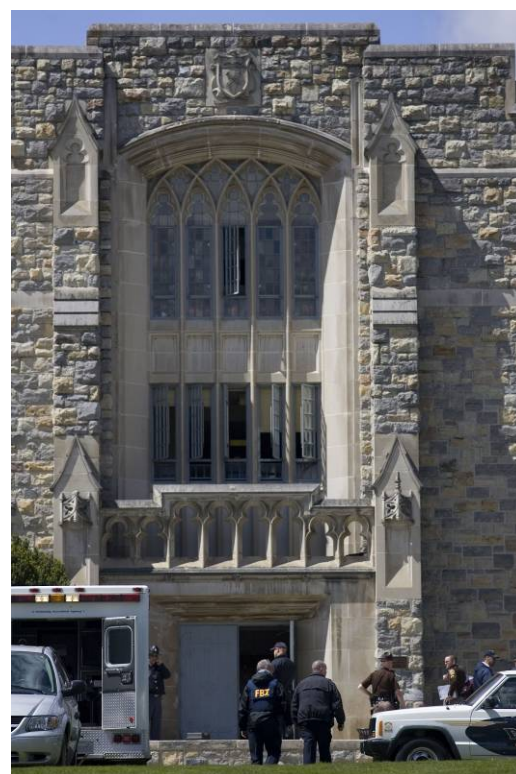
Figure 7. One of the Main Entrances to Norris Hall
