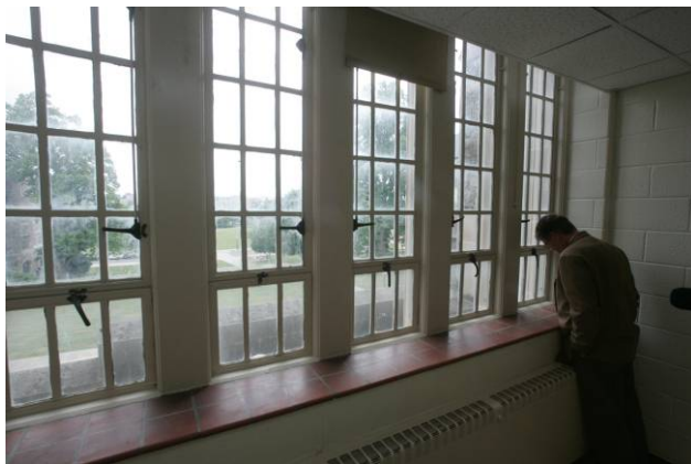
Figure 11. Typical Set of Windows in Norris Hall
